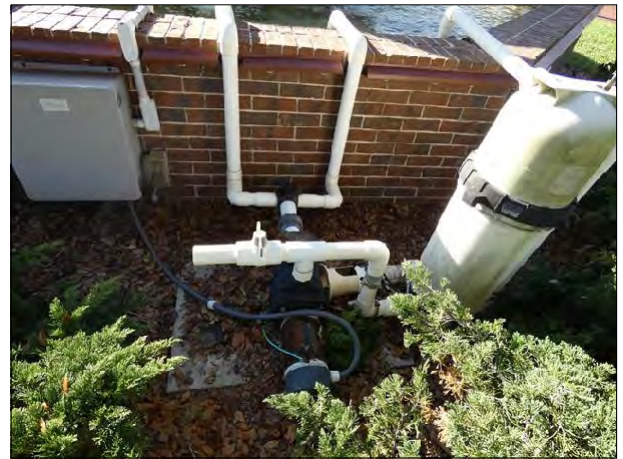
Connerton Blvd Fountain Equipment, Note Rusting Pump
