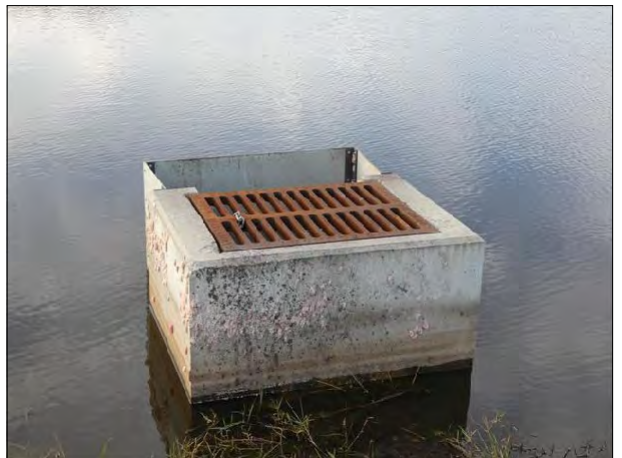
Stormwater Drainage Control Structure
